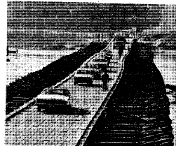
Once the engineers had the one lane float bridge in place, travel was able to resume at an almost normal pace.
