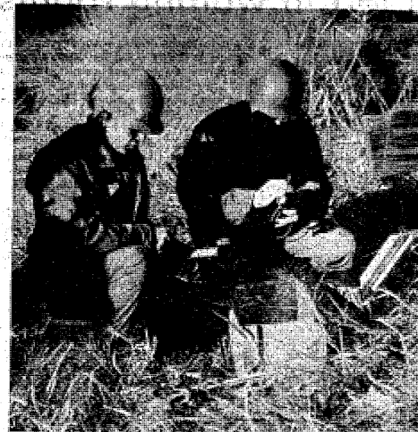
Soldiers of D Co, 20th Engr Bn (Ft. Campbell, KY) prepare sticks of the timber trussell span of the bridge. dynamite for the internal charges placed in (US Army Photo)
